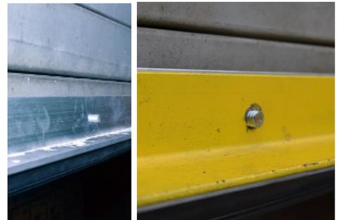
10. Fit the rubber portion of the Xcluder Roll-up Door Seal inside the roll-up door guides.
