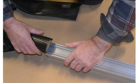
8. Install and crimp the end clips on to each end of the Xcluder Roll-up Door Seal.
