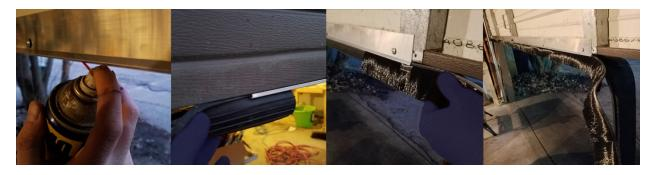
7. Take the loose retainer and cut to fit remaining space. Lubricate channels, as before. Carefully, feed the T-Rubber and Brush Seal into the retainer, pulling the retainer & seals "together", until "loose" retainer sits flush against mounted retainer:
