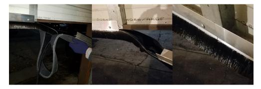
9. Cut off excess T-Rubber and Brush using heavy duty scissors (shears).
