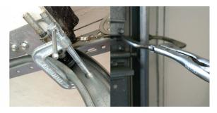
1A. Measure door thickness, ensuring you have the appropriate retainer. X2s come in 3 sizes for garage doors: 13/8", 1 3/4", and 2". 1B. Measure the width of your door to determine you have the correct kit. Kits are available for standard width garage doors: 8', 12', and 16'. If your garage door does not match these sizes order the next wider door.
